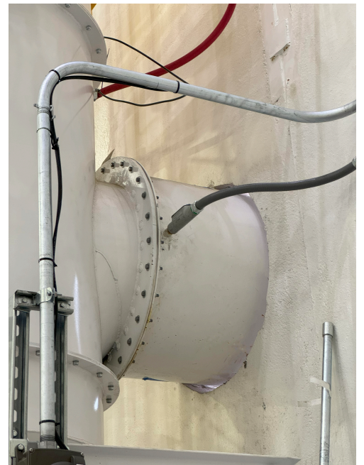
Explosion Vent ducted outdoors.
